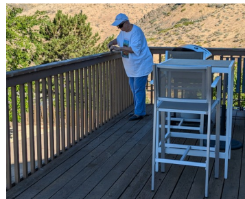
Applying wood preservative to our deck.
